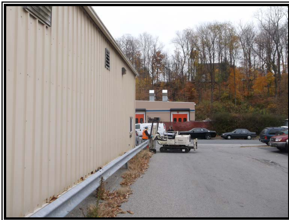
Photograph taken during installation of GB-3
