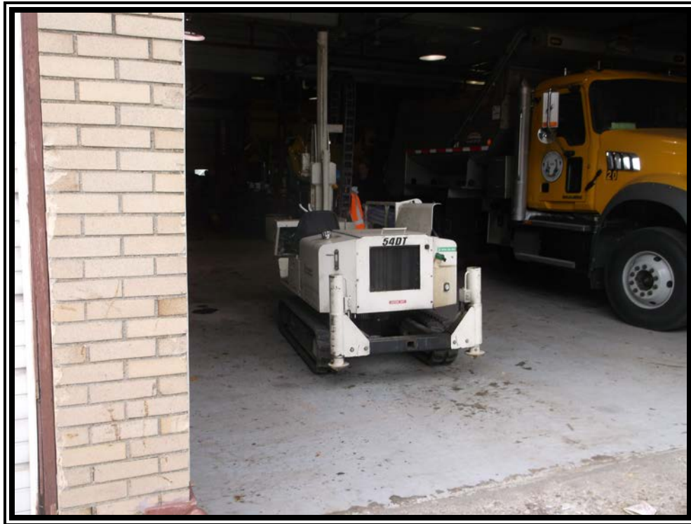
Photograph taken during installation of GB-1
